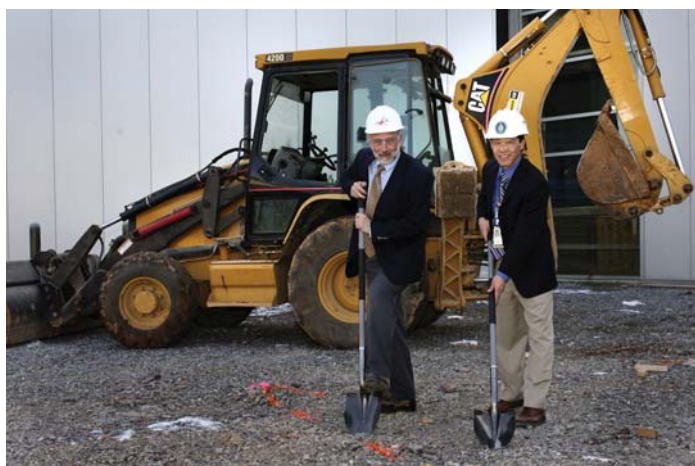
Physics Professor Geoff Greene (left) and David Arakawa of the Department of Energy break ground at the SNS for a building to house the neutron electric dipole moment experiment.
